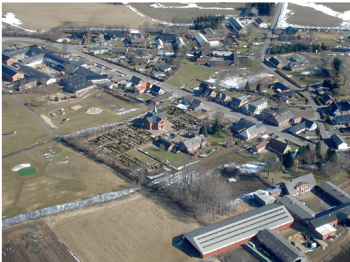
Fig. 2. Luftfoto af kirken set fra sydvest, 2013. Bredsten Lokalkiv. – Aerial photo of the church seen from the south west.
