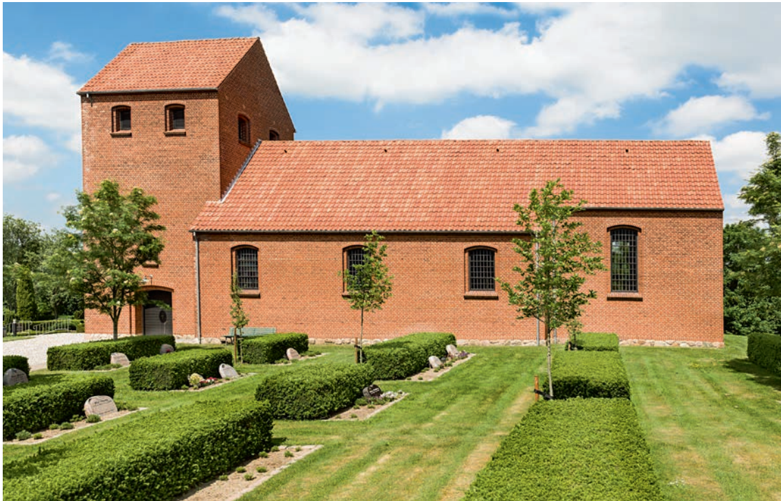
Fig. 1. Kirken set fra syd. Foto Arnold Mikkelsen 2015. – The church seen from the south.
