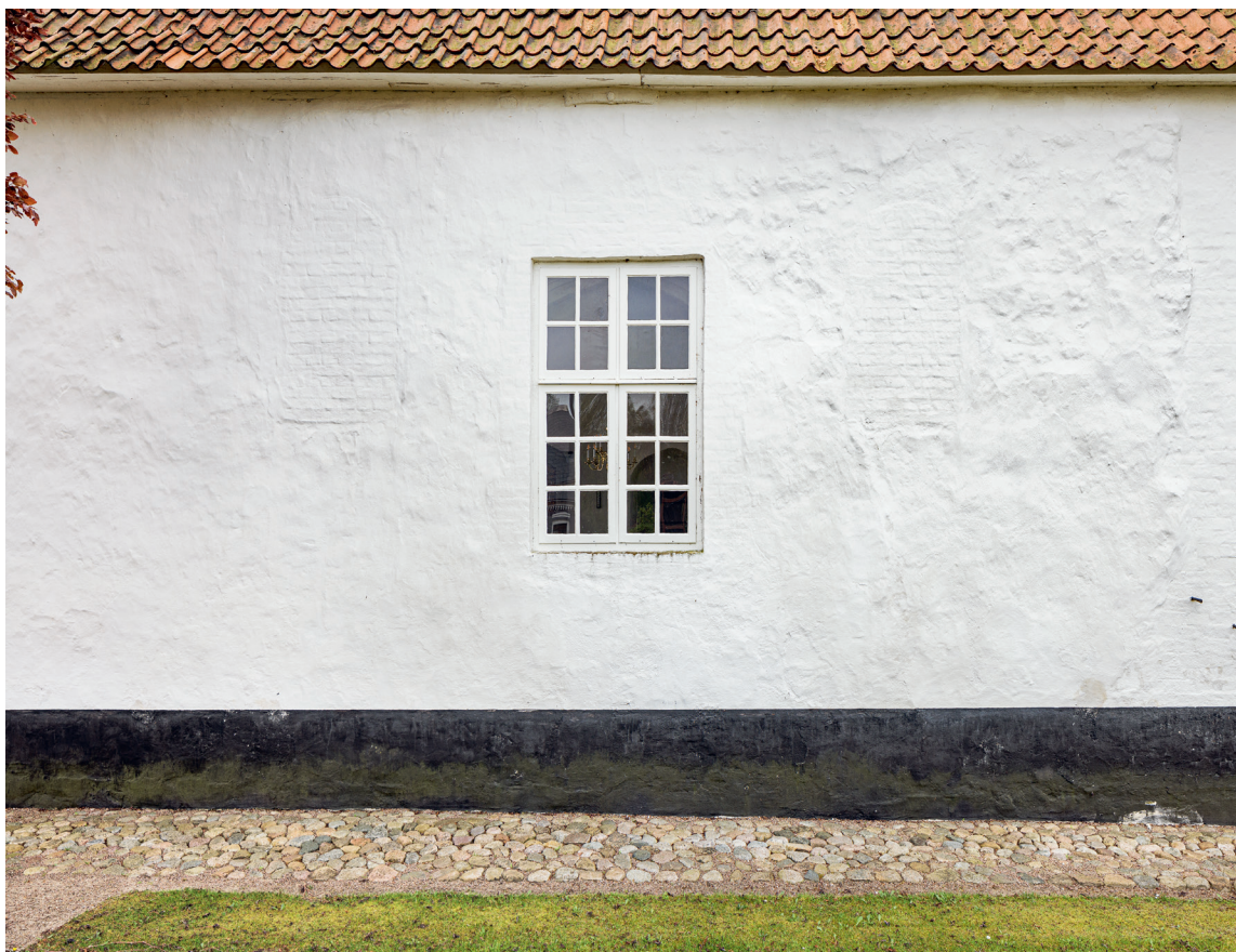
Fig. 130. Vindue fra 1864 samt to tilmurede, romanske \dagger vinduer i skibets nordmur (s. 3997 og 3982). Under vinduet fandtes den nu forsvundne \dagger norddør (s. 3981). Foto Arnold Mikkelsen 2023. – Window from 1864 as well as two bricked-up Romanesque \dagger windows in the north wall of the nave. Below the window was the now absent north \dagger door.
