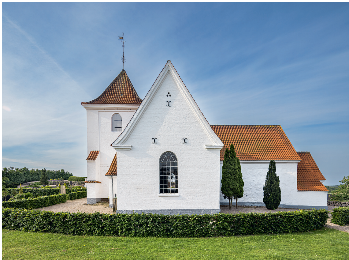
Fig. 11. Ydre set fra nord. Foto Arnold Mikkelsen 2021. – Exterior seen from the north.
