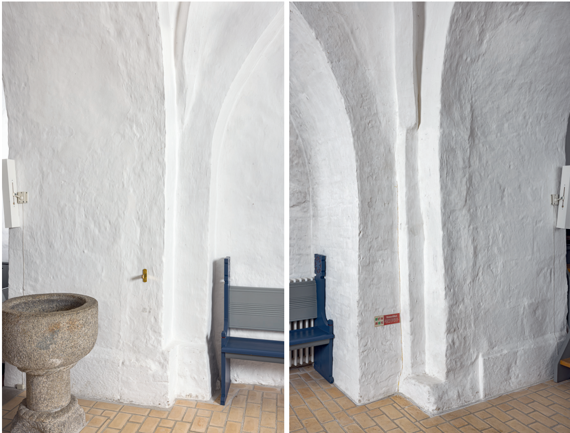
Fig. 22-23. 22. Triumfbuens nordre vange set fra syd, samt det ældre \dagger korhvælvs nordvestre hjørnepille (s. 6313). 23. Det udvidede kors sydvestre hjørne med hvælvpille og korbuens søndre vange (s. 6313). Foto Arnold Mikkelsen 2021. – 22. Northern side member of the chancel arch, seen from the south, as well as the north west corner pier of the older \dagger vault. 23. The south-west corner of the extended chancel with a vault pier and the southern side member of the chancel arch.
