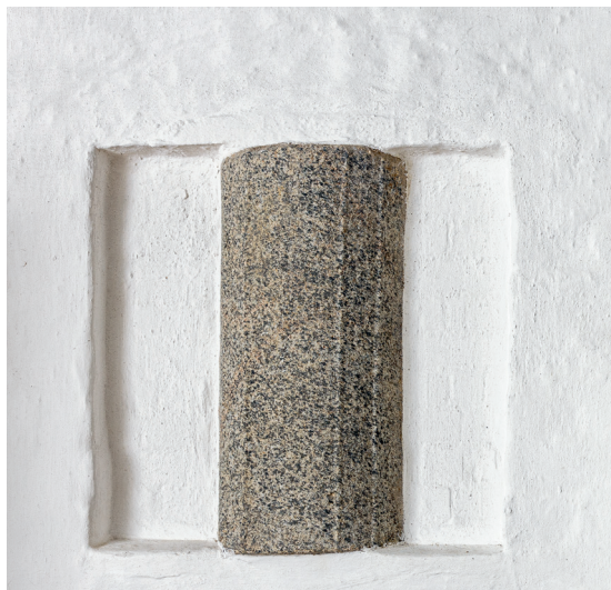
Fig. 101. Sojletromle (s. 6386, note 54), indmuret i våbenhuset vestmur. Foto Arnold Mikkelsen 2021. – Column drum walled into the west wall of the porch.
