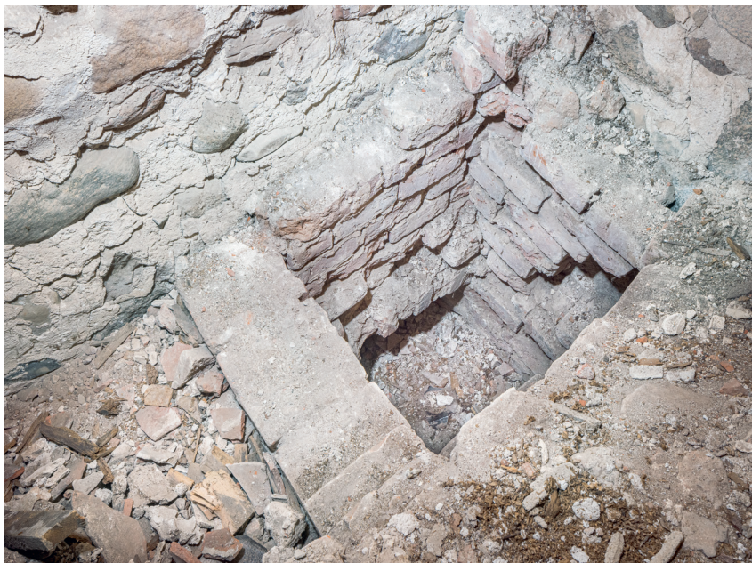
Fig. 41. Muret skakt (s. 6331) i sakristiets sydvsthjørne, set fra sakristiets loftsrum. Foto Arnold Mikkelsen 2022. – Masonry shaft in the south west corner of the sacristy, seen from the loft of the sacristy.
