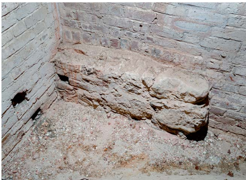
Fig. 58. Rest af skibets romanske, vestre gavltrekant set fra tårnets mellemstokværk (s. 4905). Foto Arnold Mikkelsen 2018. – Remains of the Romanesque western pediment of the nave seen from the middle floor of the tower.
