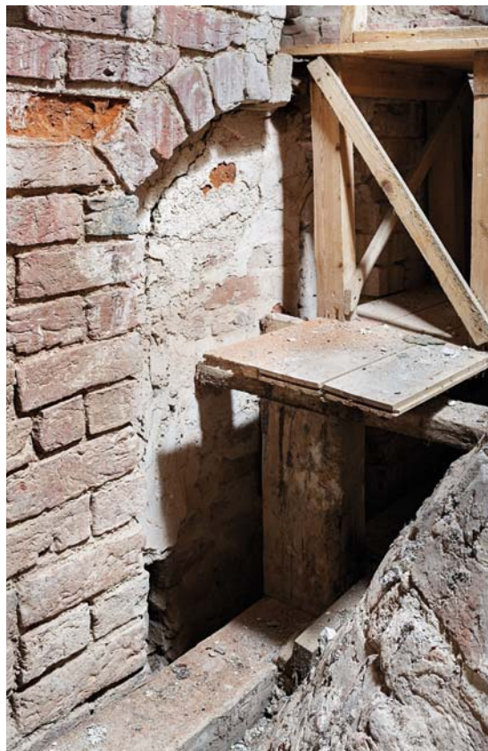
Fig. 7. Det søndre, blændede vindue i tårnets østmur set fra skibets loft (s. 3013). Foto Arnold Mikkelsen 2014. – Southern bricked-up window in the east wall of the tower seen from the ceiling of the nave.
