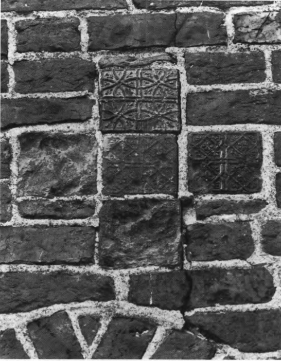
Fig. 6. Gulvfliser fra o. 1250-1300, indmuret i korgavlen over vinduet (s. 1090, 1092). NE fot. 1979. - Floor tiles c. 1250-1300 built into the chancel gable above the window.
