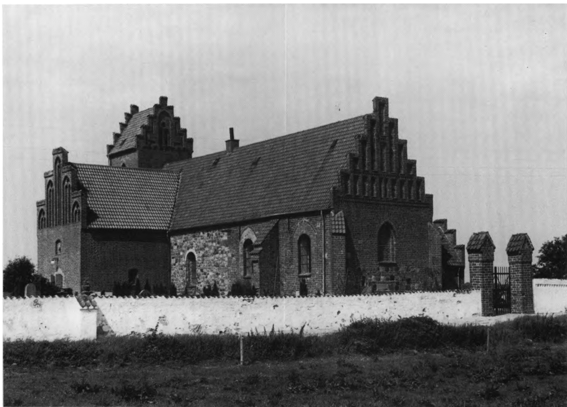
Fig. 1. Kirken set fra sydøst. NJP fot. 1979. - The church seen from the south-east.
