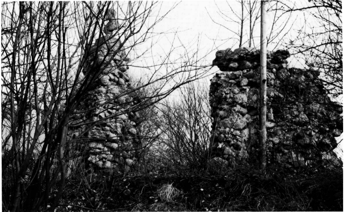
Fig. 1. Ruinen set fra sydvest. KdeFL fot. 1984. - The ruin seen from south-west.
