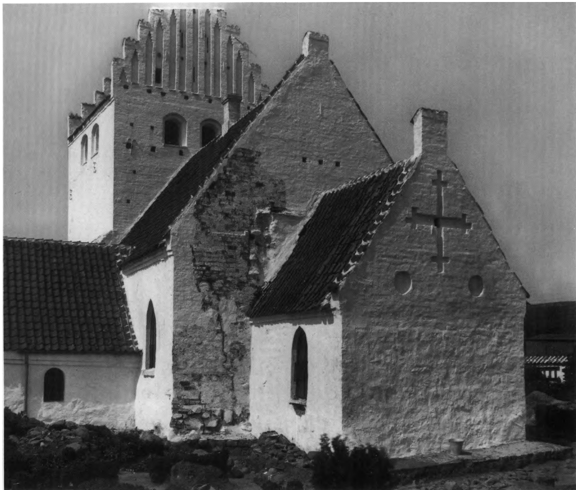
Fig. 9. †Kor og †triumfmur set fra sydøst. Forneden to skifter murværk fra rundskibets østfacade (s. 2519); over korets sydmur spor af det oprindelige andet stokværk. Kai Uldall fot. 1925. - †Chancel and †east wall of the nave seen from the south-east. Below, two courses of masonry from the east facade of the round nave; above the south wall of the chancel are traces of the original second storey.
