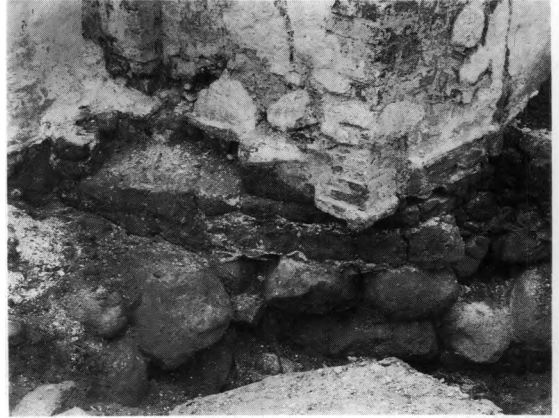
Fig. 12. Rest af rundkirkemur i nordre hjørne mellem kor og triumfmur (s. 2519); i forgrunden til venstre fundament af planlagt korudvidelse (s. 2529). Kai Uldall fot. 1925. - Traces of masonry from the round church in the north corner between chancel and east wall of the nave; in the foreground, on the left, the foundation of proposed enlargement of the chancel.
