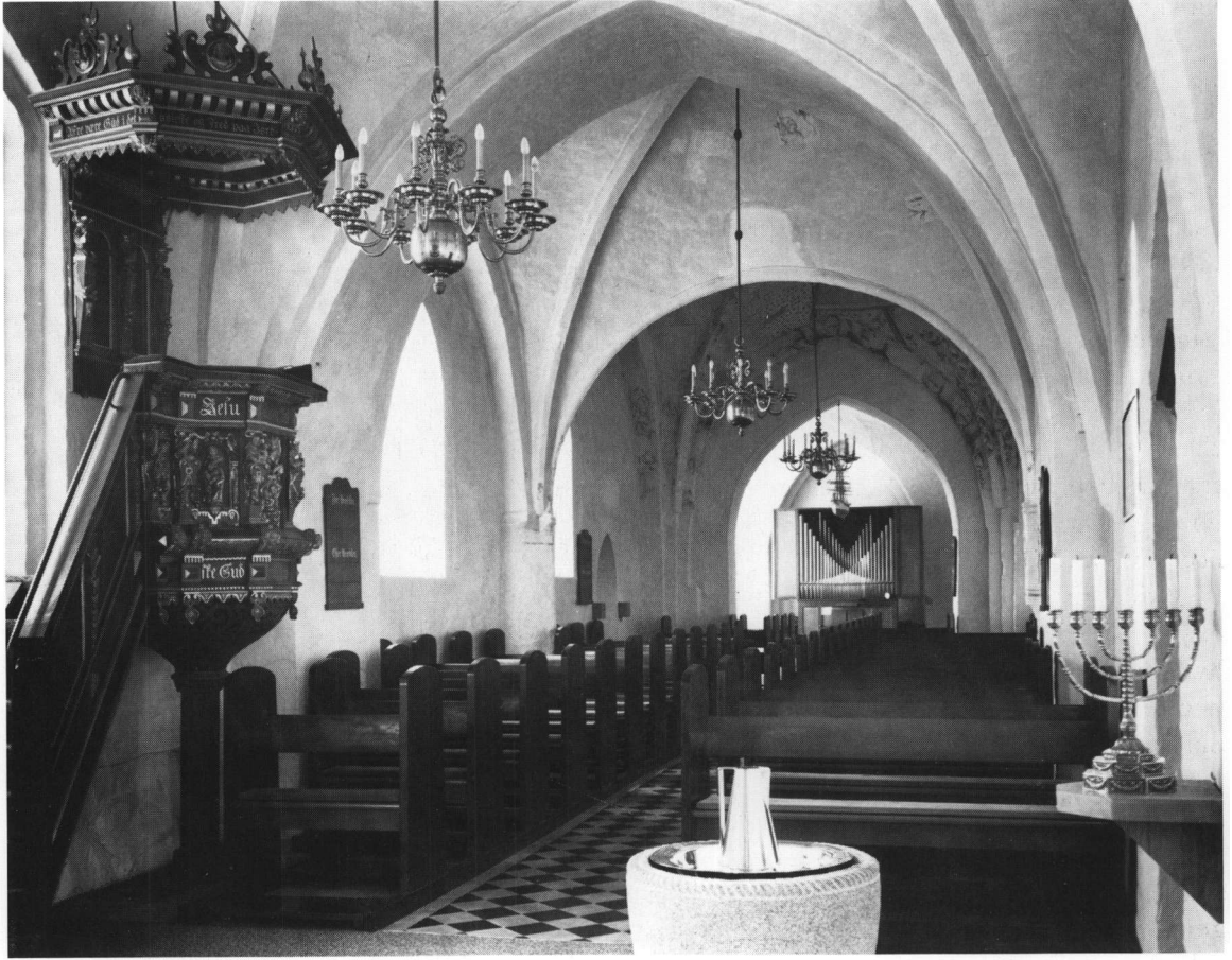
Fig. 7. Indre, set mod vest. NE fot. 1985. - Interior to the west.
