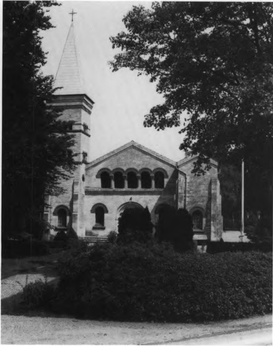
Fig. 1. Ydre, set fra vest. HJ fot. 1984. - Exterior seen from the west.
