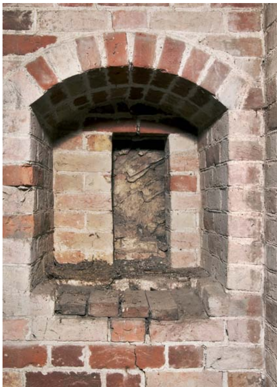
Fig. 11. Glug i tårnets østmur i 1. mellemstokværk (s. 1923–24). I bunden af gluggen ses 'bagsiden' af midterskibets vestre skjoldbue. Foto Arnold Mikkelsen 2007. – Peephole in the tower's east side 2. floor wall. The "rear" of the middle aisle's western supporting arch is evident through the base of the peephole.
